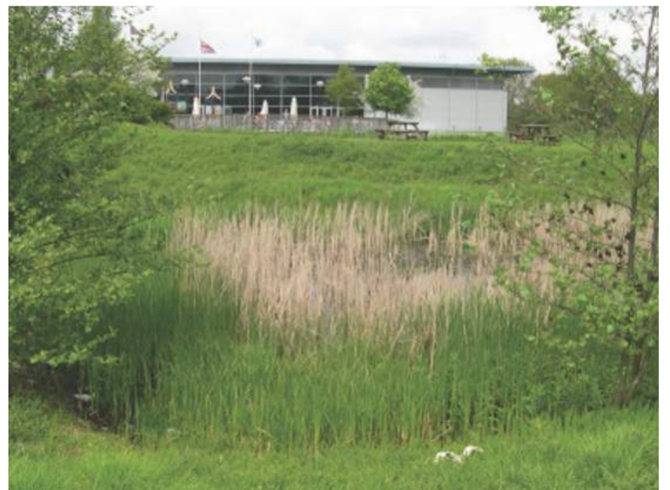
SuDS Pond/Wetland, Hopwood Service Area, M42
