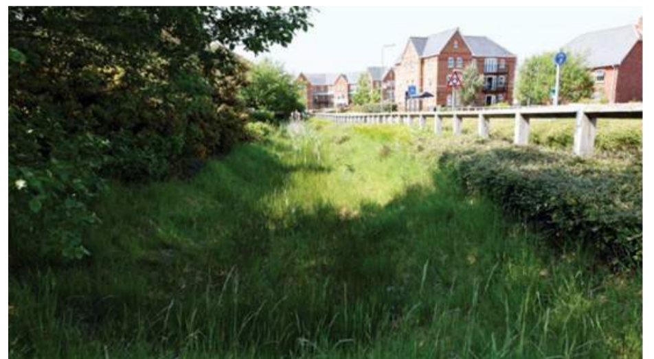
Roadside Swale, Elvetham Heath, East Hampshire
